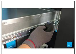
Release second lever inside the Rack and continue sliding the G5000 Controller into the Rack
